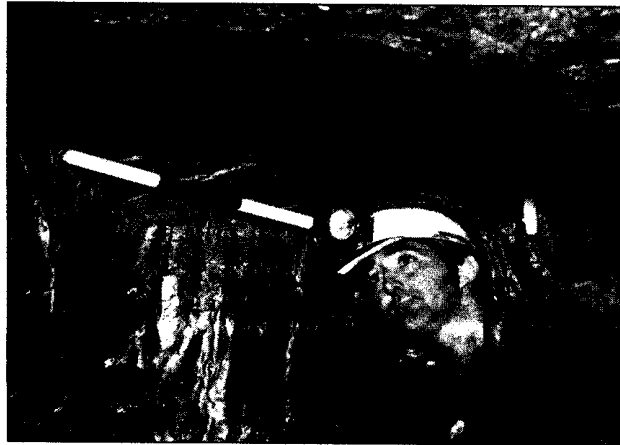
FIGURE 23.1 Large kettle bottom in an underground coal mine (photo by F. Chase)
