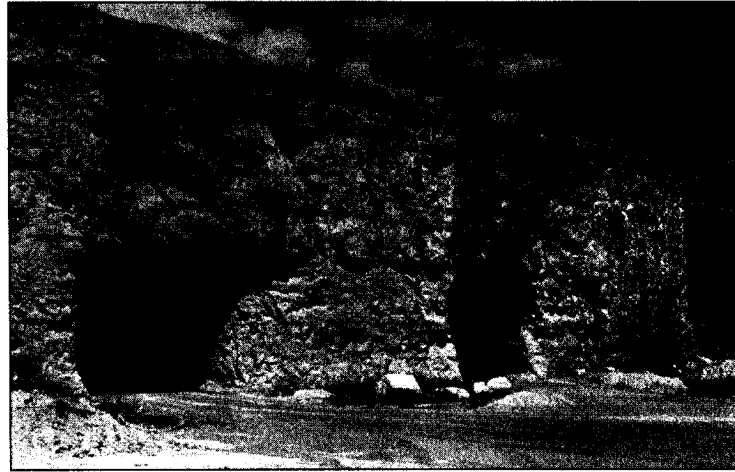
FIGURE 23.11 Smooth roof line produced by a persistent bedding plane lamination within the roof rock beam
