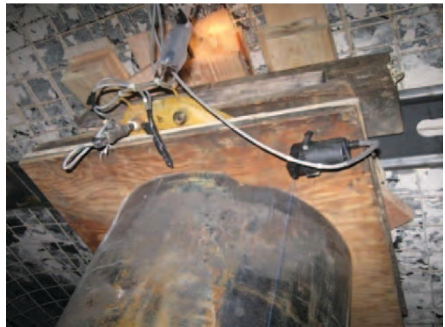
Figure 4. Load cell and displacement transducer installed on a CAN.
