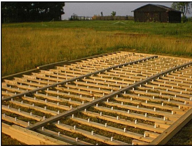
Figure 3.—Completed wood frame with PVC pipe holders.
