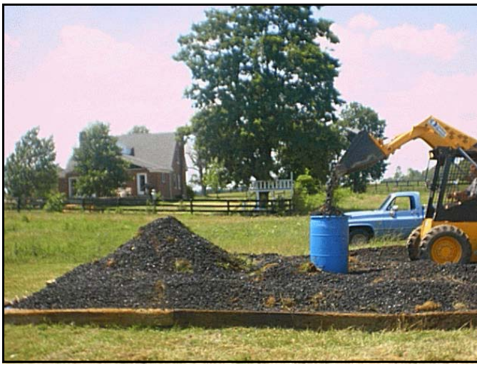
Figure 7.—Second perforated plastic barrel being covered with coal.
