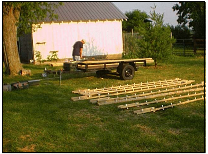
Figure 2.—Assembly of 1.3 cm (0.5 in) in diameter PVC pipe inserted into 2- by 4-in studs.
