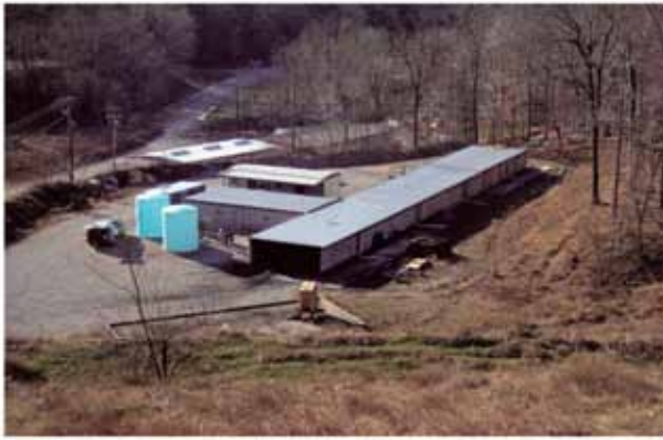
Figure 1 — Fire Suppression Facility.
