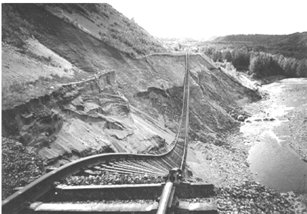
Figure 6. Rail track demolished by a slope failure.
