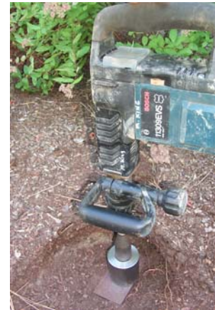
Figure 10—Demolition hammer vibration source
