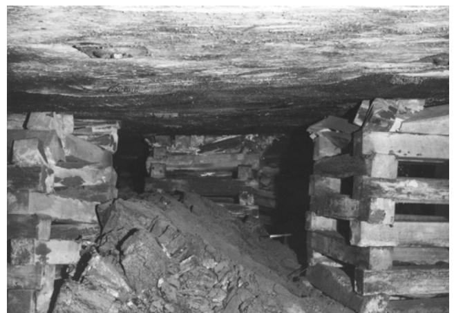
Figure 2. Excessive pillar line floor heave.
