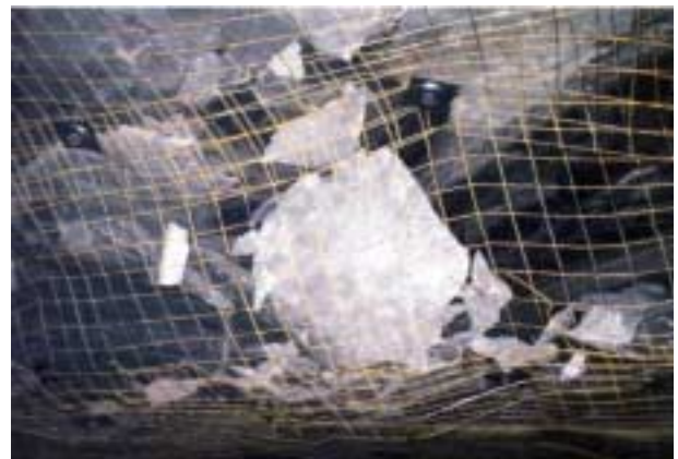
Figure 1. Roof Screen effectively maintaining weak roof skin.
