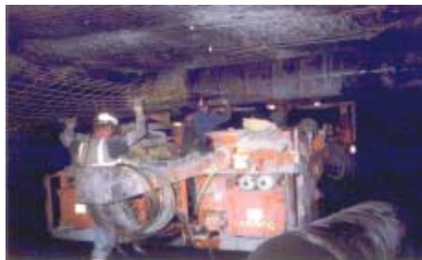
Figure 6. Roof bolting operators handling roof screen on a walk-through bolting machine.
