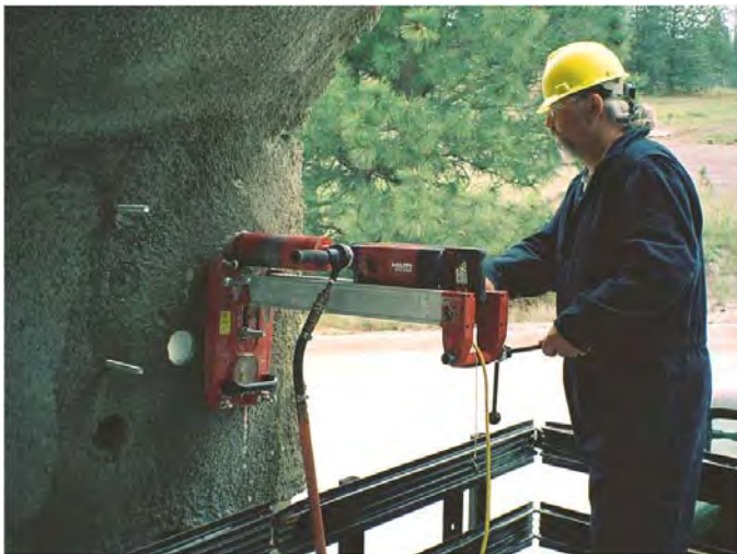
Figure 10. Drilling an adhesion test core on a vertical surface.
