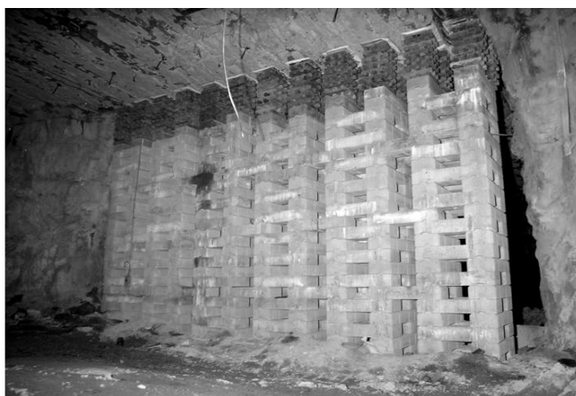
Figure 6. Crib wall to protect the secondary escapeway.
