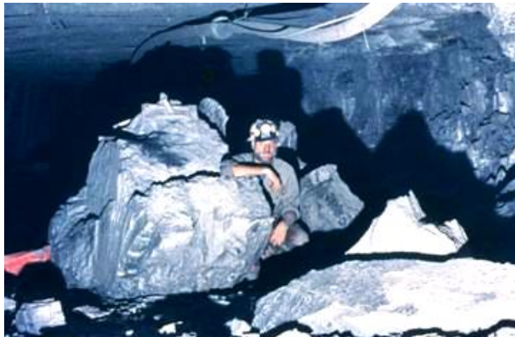
Figure 5. A rib fall involving large blocks of rock and coal.
