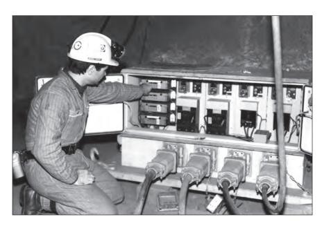
Figure 6. Sensitive AC GFR's installed in Safety Research Coal Mine
