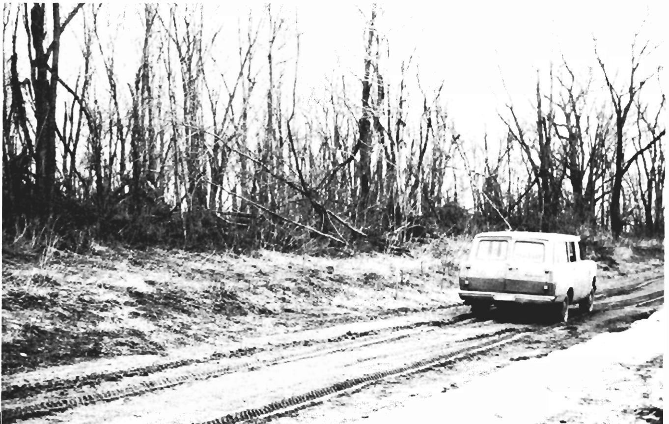
FIGURE 3. - Drilling site before preparation. Photograph taken March 1978, view is east.
