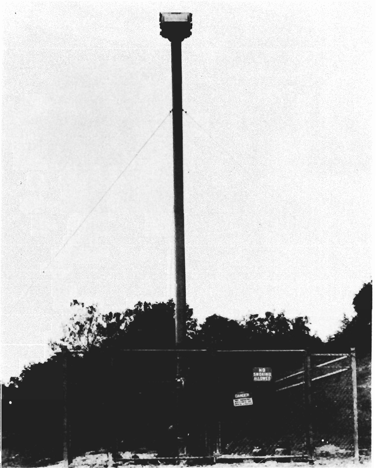
FIGURE 5. - Surface venting facility.
