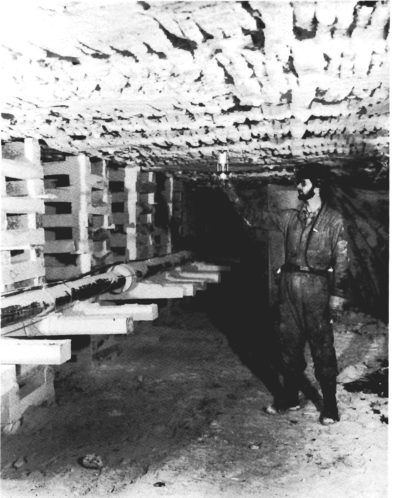
FIGURE 3. - Steel pipeline and cribbing blocks.
