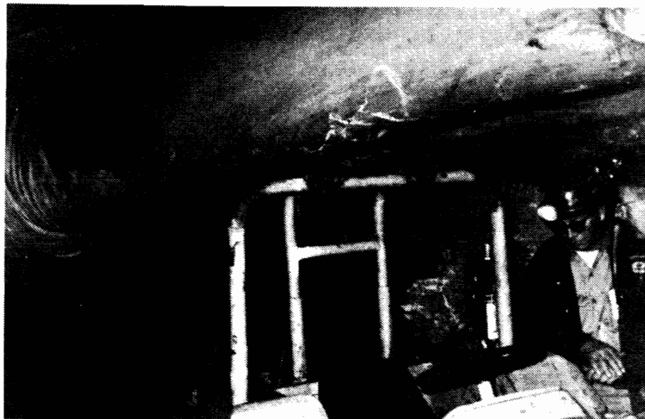
Figure 4-31. Underground Mine Canopy Clearance Problems
