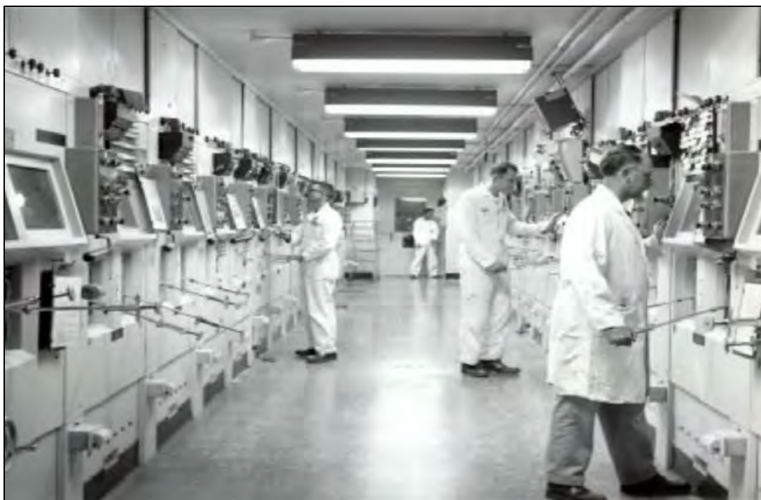
Figure 5-26: Shielded Glove Boxes in the Remote Analytical Facility
