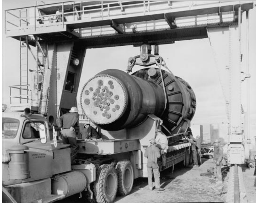
Figure 5-42: ETR Reactor Vessel Arriving at CFA Gantry Crane in 1956
