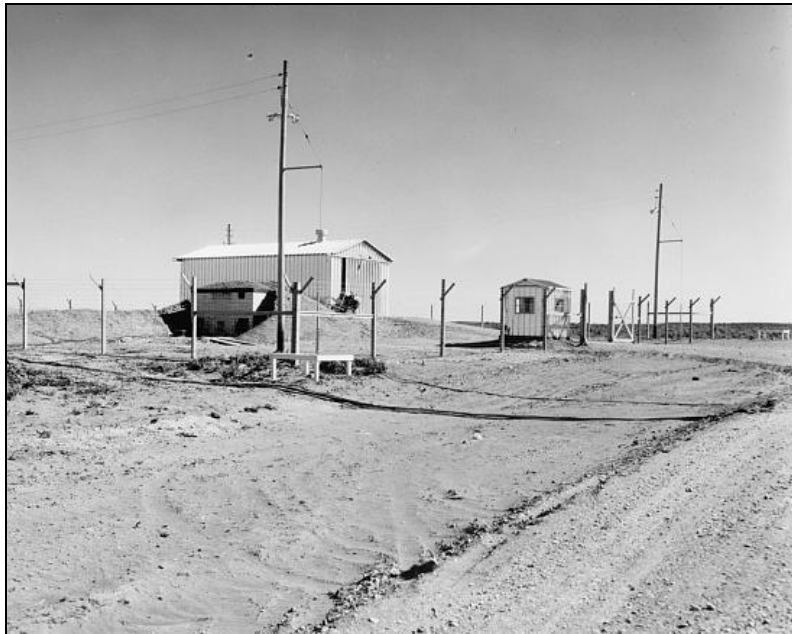
Figure 5-40: The SPERT-I Facility
