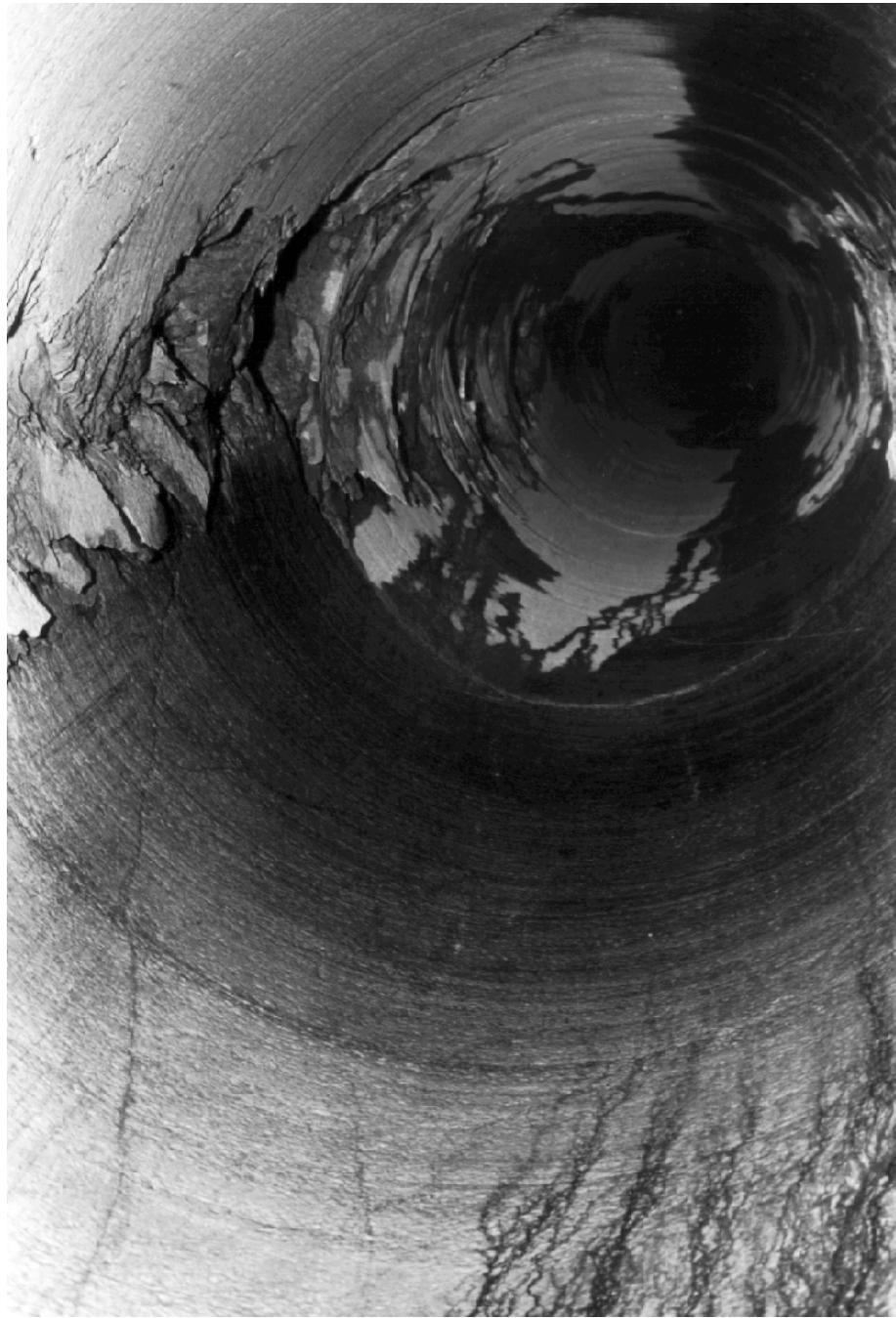
Raise bore breakouts, 7300 level, Star Mine.
