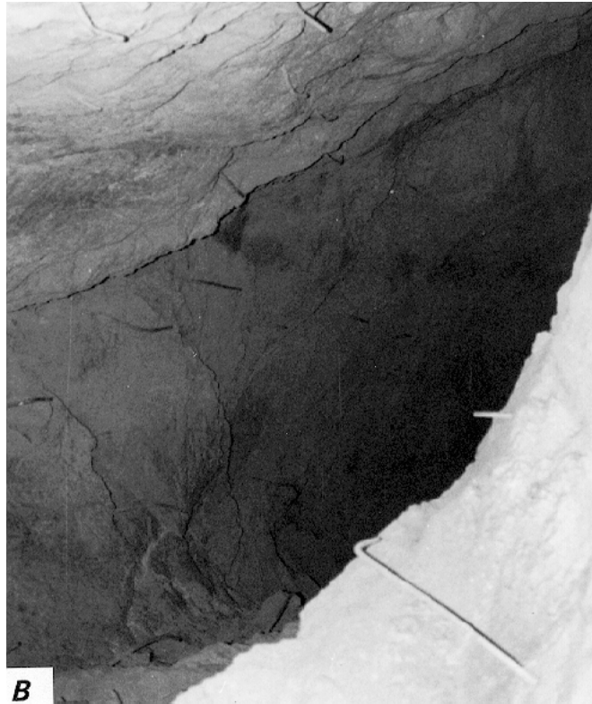
Breakouts observed in Silver shaft ore passes on 5100 level. A, Plan view. Circle (dotted line) indicates original shape of ore pass, while ellipse (solid line) indicates final shape after breakouts occurred. B, Breakout as observed looking down north ore pass.
