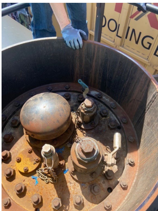
Figure A5. Inside the valve housing on top of the tank railcar containing hazardous materials. Photo by NIOSH.
