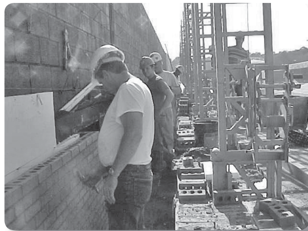
Solution: Masons finish top course on split-level adjustable scaffolding
