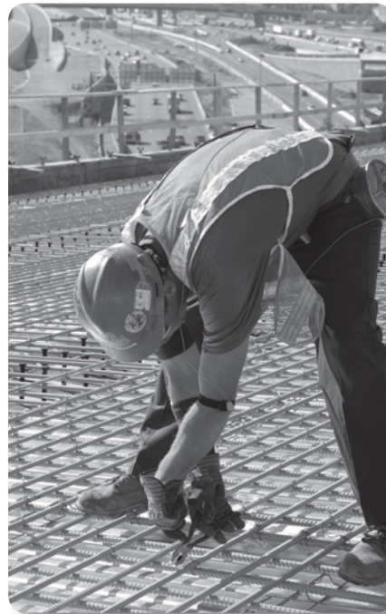
Problem: Tying rebar by hand
