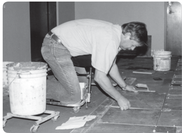
Solution: Laying tile with kneeling creeper
