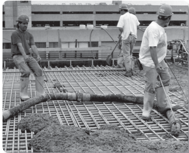
Problem: Pulling concrete hose without skid plate
