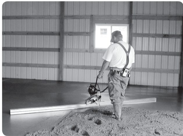
Solution: Motorized screeding
