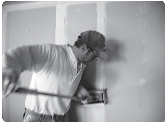
Problem: Hand drywall finishing with mudbox
