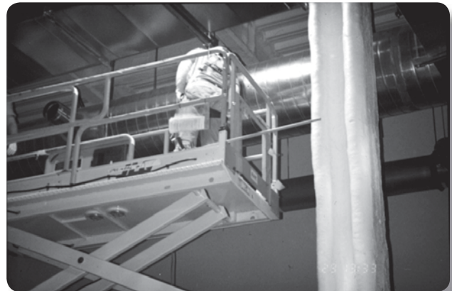
Person-lifts provide stable platforms for overhead work and eliminate handling of ladders and scaffolding
