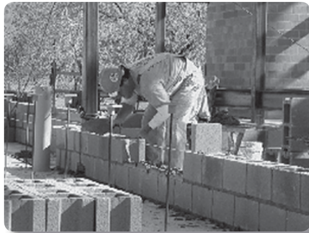
Problem: Laying standard concrete block
