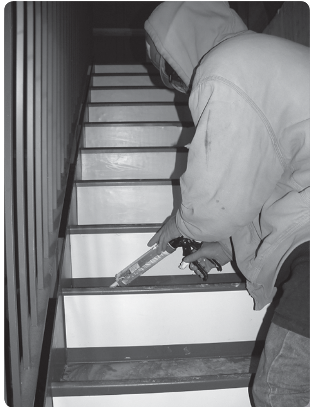
Problem: Manually squeezing caulking gun
