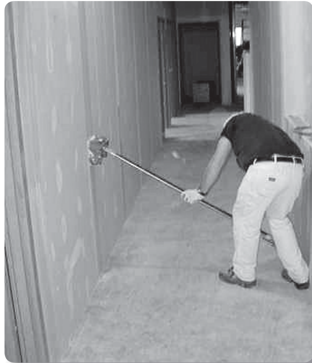
Problem: Hand drywall finishing with mudbox
