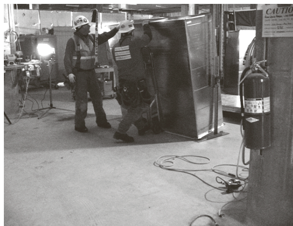
Figure 2-5.9. Removing the completed duct
