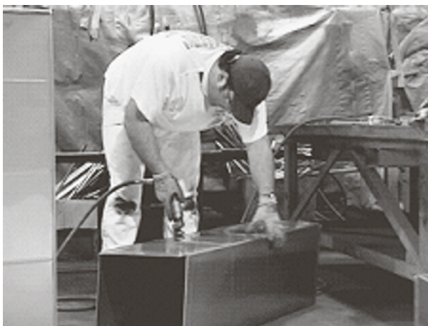
Figure 1-1.10. Using the floor as a workbench
