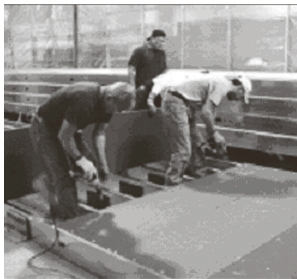
Figure 3-2.2. Modularizing sheet rock
