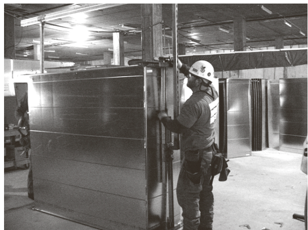
Figure 2-5.4. Setting up the clamp
