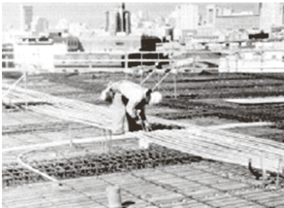
Figure 2-1.3. Worker installing pipe on deck
