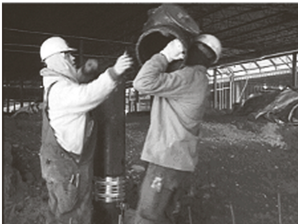
Figure 1-1.9. Carrying or lifting heavy materials
