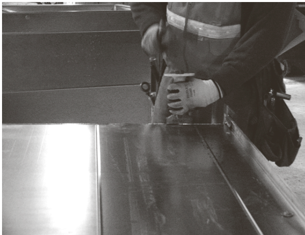
Figure 2-5.6. Setting a Pittsburgh seam
