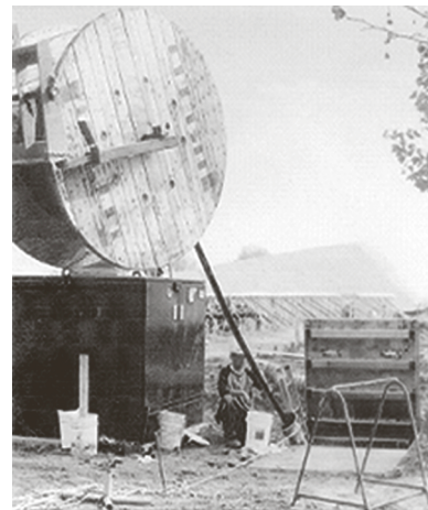
Figure 2-1.6. Elevated reel to assist installation
