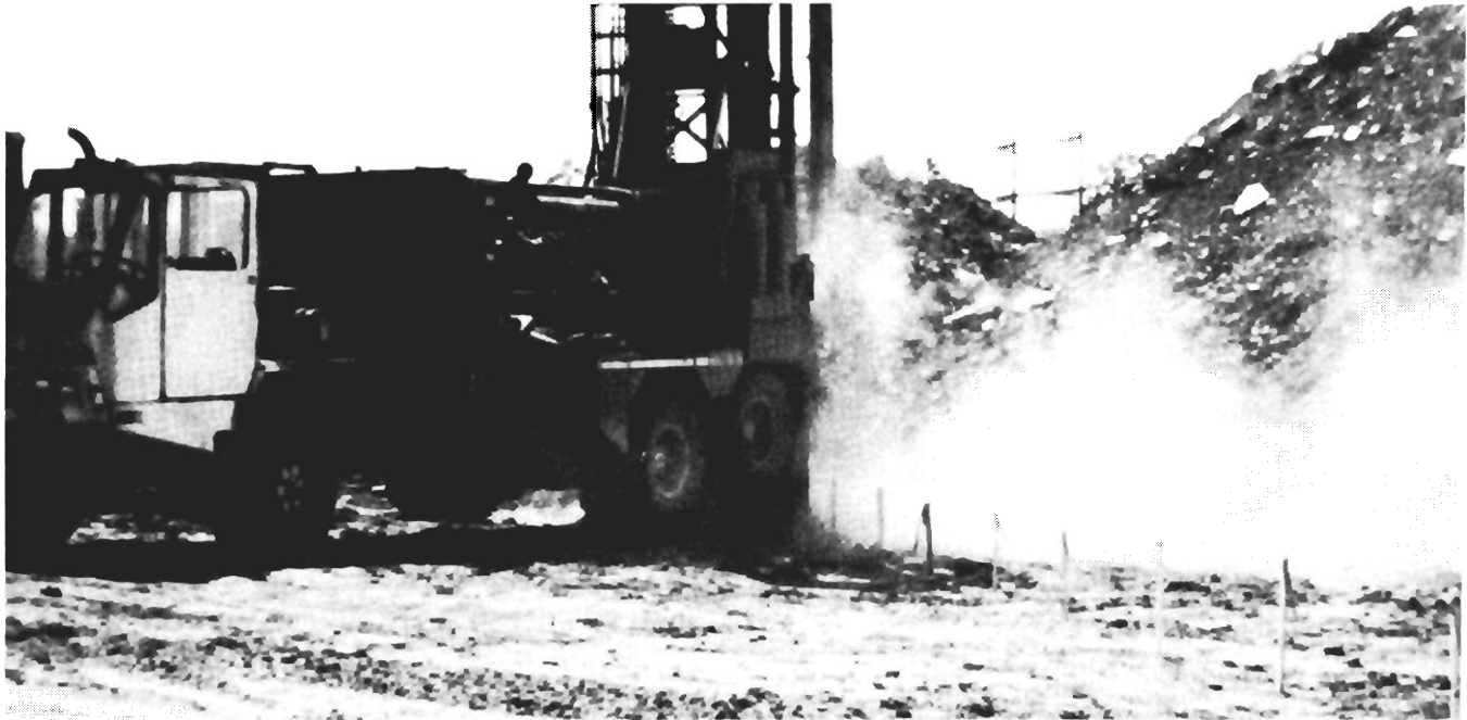
FIGURE 7. - Test holes being drilled.
