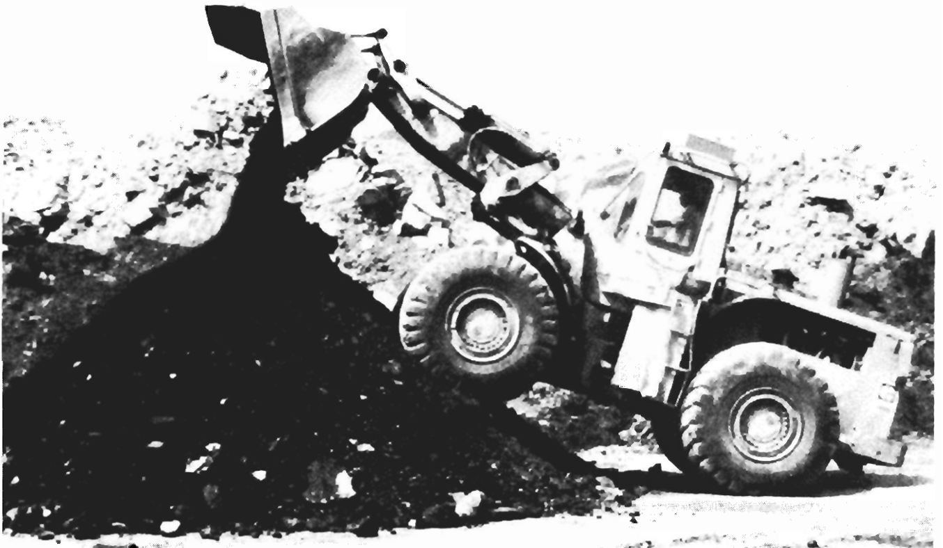
FIGURE 6. - Overburden being placed over transmitter.
