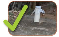
Septic tank ventilation pipe with screen mesh
