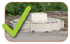
Septic tank sealed with PVC cap
