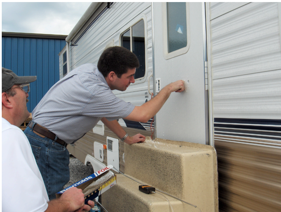
Figure 1. Preparation for indoor sampling in a THU. Half inch holes were drilled into the THU door for insertion of \frac{1}{4} " stainless steel sampling tubes. A sampling tube and sample pump are seen in the foreground.
