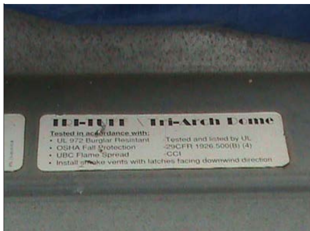
Exhibit 6. The identification tab on the skylight the victim fell through.
