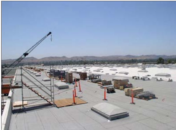
Exhibit 1. The rooftop looking south.
