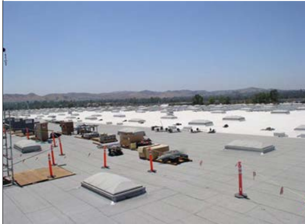
Exhibit 2. The rooftop looking west.
