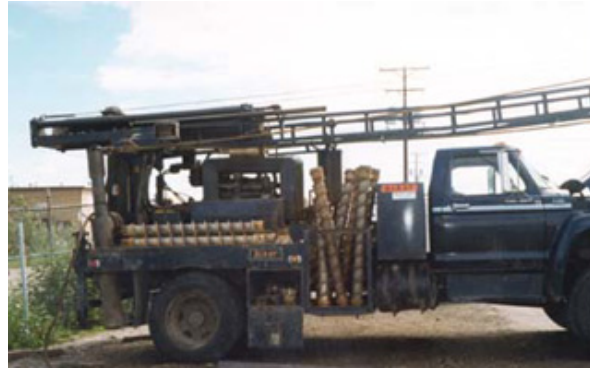
Figure 2b. View of drill rig, passenger side
